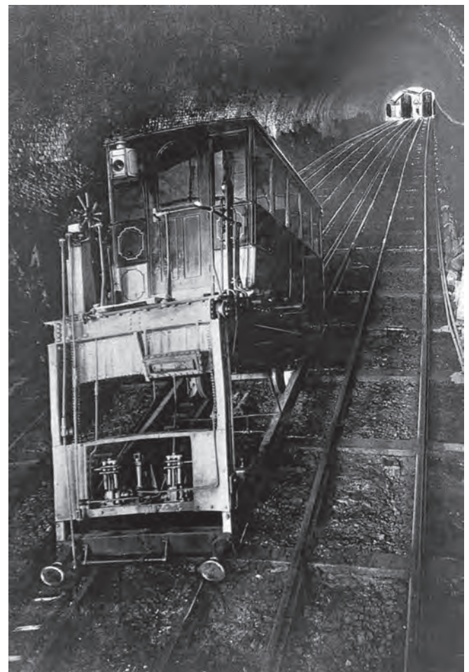
Each car consisted of an upper passenger section, with a triangular chassis angled to suit the gradient of the tunnel. Each car could accommodate 18 seated passengers and had sliding doors at either end
